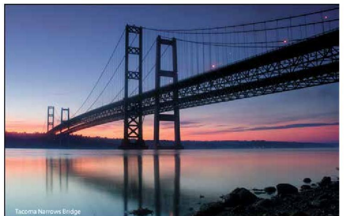
Tacoma Narrows Bridge
