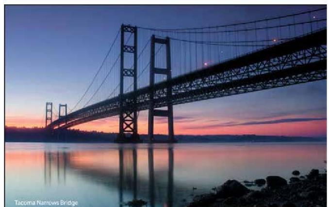
Tacoma Narrows Bridge
